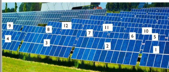
AGC control based on real time monitoring of reference inverters (un-controlled inverters) where controlled inverters only will respond for AGC signals.
